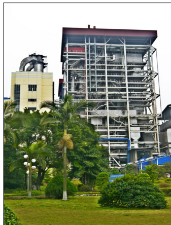
Heshan power plant
