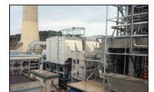
Shajiao C power plant
